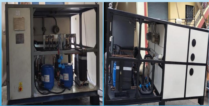
Refurbishments of Old/Unused Environmental Chambers
